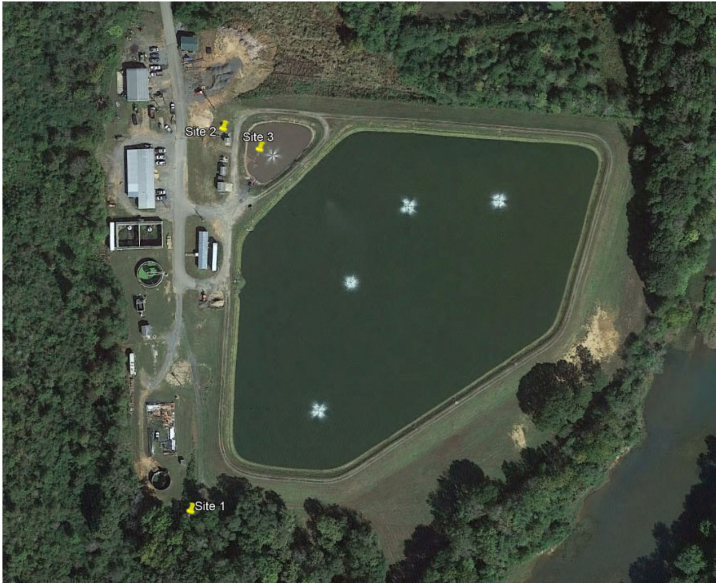
Figure 3: Sampling Site Locations at WWTP
